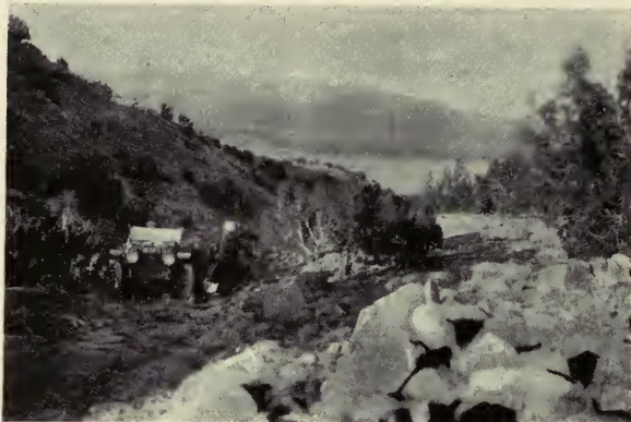
At many a place in the rugged country of Colorado and New Mexico, where now the touring motorist finds well constructed highways, the pathfinder struggled up narrow defiles, steep and rocky
